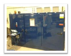
The purpose of this project was to provide the electrical drawings, PLC/HMI software design, panel built, and commissioning for a new spiral freezer control system. The objective was to provide the customer with a controls solution to operate the spiral freezer, including a clean-in-place system, steam pasteurization system, and full refrigeration and defrost control.
